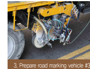
3. Prepare road marking vehicle #3
