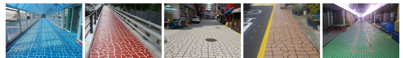
Seobinggo station overpass, Seoul Bucheon station overpass, Gyeonggi-do Uijeongbu specific street, Gyeonggi-do Seodaemun safe footpath, Seoul Gyeongin market, Incheon
