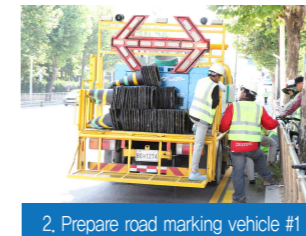
2. Prepare road marking vehicle #1
